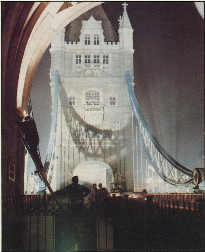
Final adjustment of luminaires.
