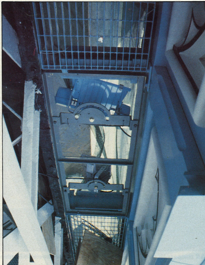
Floor trap in high level walkway houses the road lighting.
