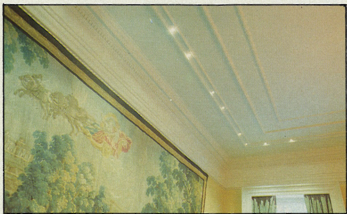
Fibre optic spotlights recessed between ceiling moulding at Polly Peck International.
