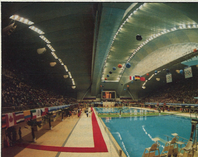
Metal halide lamp installation in the swimming hall.
