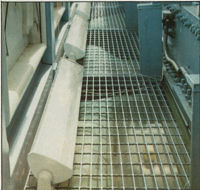
Fluorescent lamps at high walkway level illuminate the girderwork.
