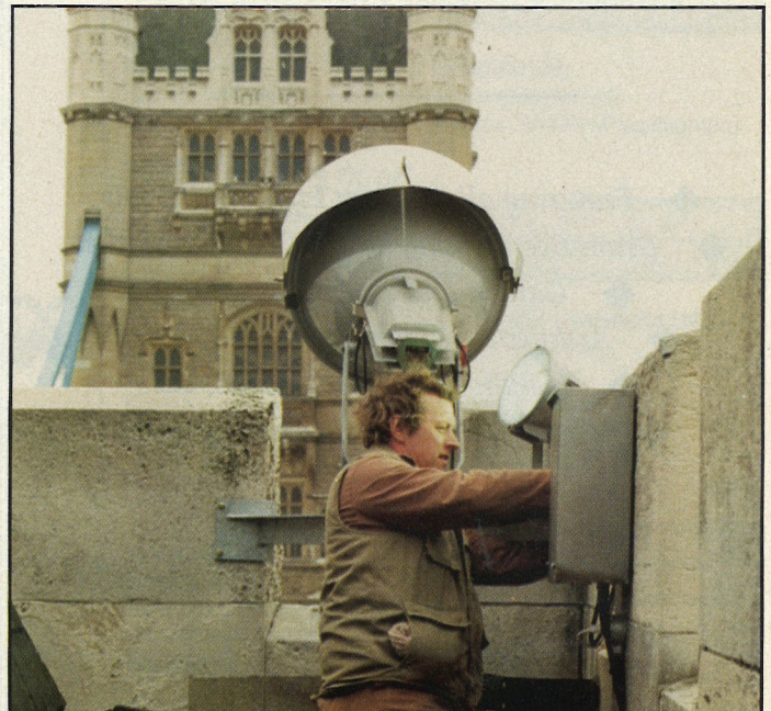
Mounting control gear for one of the floodlights to the main tower.
